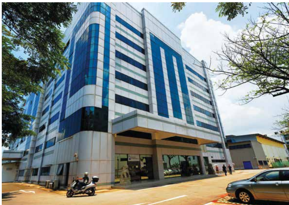
Light Industrial Building, 26 Woodlands Loop
