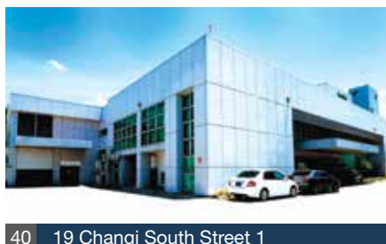
40 19 Changi South Street 1
