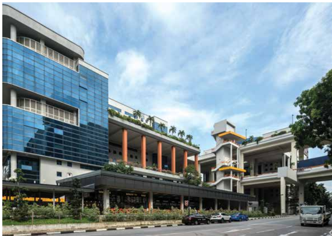
Stack-up/Ramp-up Buildings, Woodlands Spectrum
