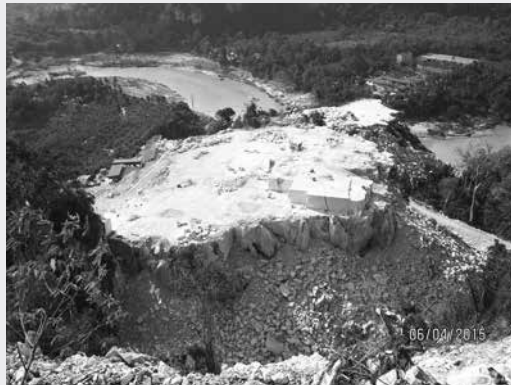
Figure 4-3; Production platform in Hill 2B
