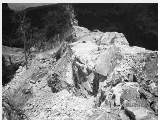
Figure 4-1; Creating access at Hill 1
