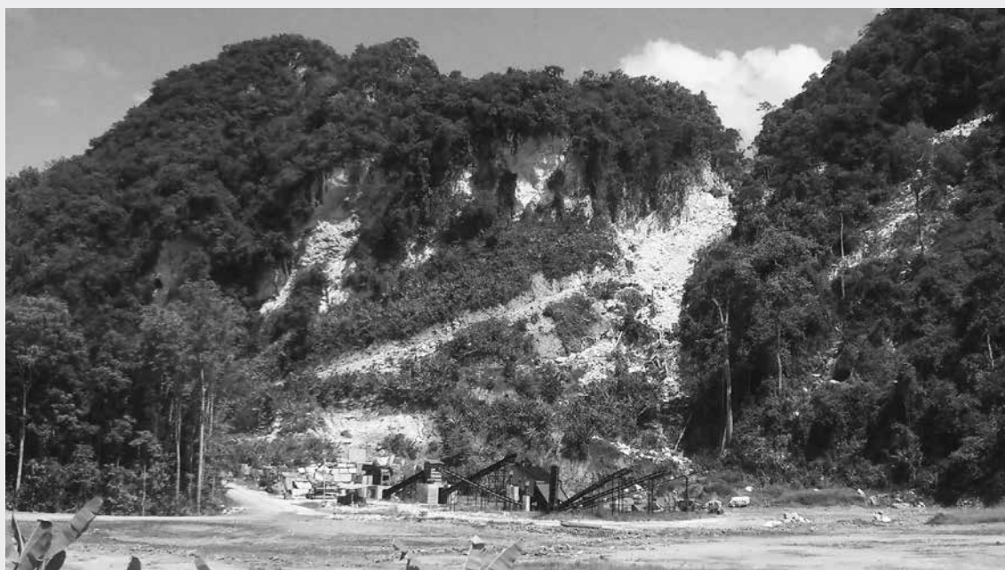
Figure 2-2; Hill 2A looking to the south from site entrance – note crushing plant in foreground
