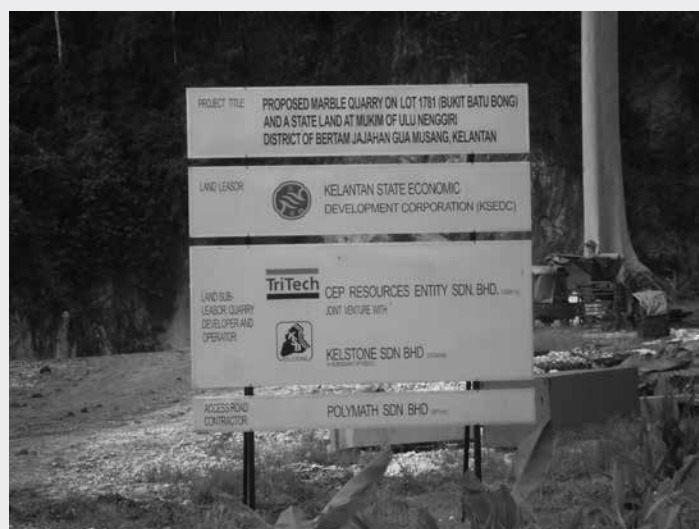
Figure 1-1; Site Entrance at the Kelantan Marble Project
