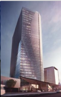
311 Spencer Street Melbourne (50% interest) -Under construction-
