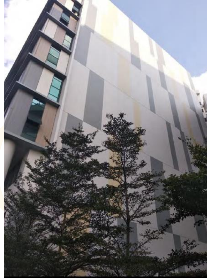
Façade re-painting and cleaning works
