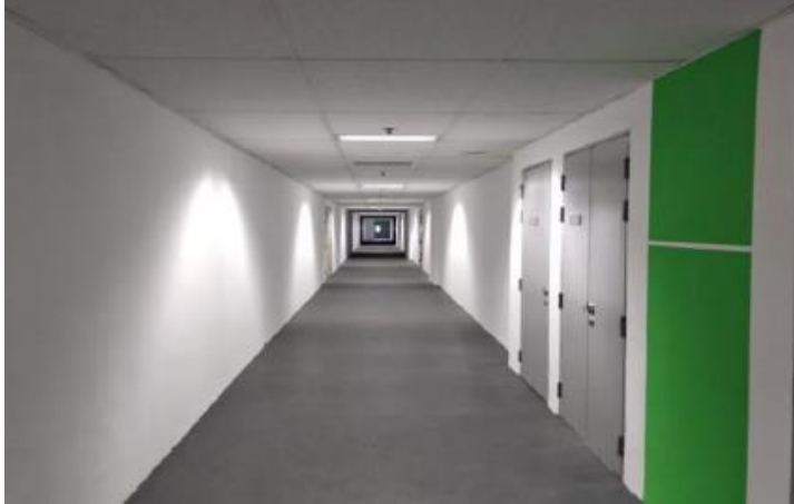
Floor finishes at common corridors
