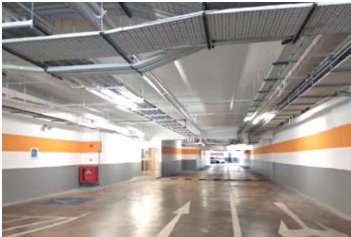
Carpark re-painting and cleaning
