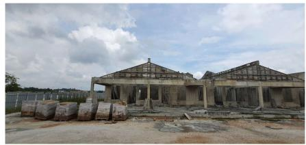
Block 3A/B: Gable wall formwork installation in progress
