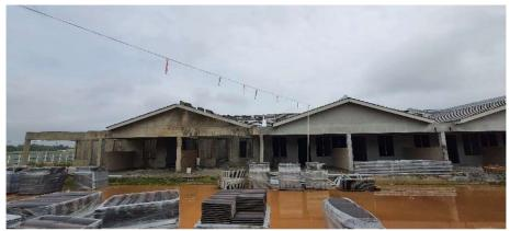
Block 2A: Roof tiles laying in progress, external skim-coating in progress
