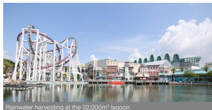
Rainwater harvesting at the 32,000m³ lagoon
