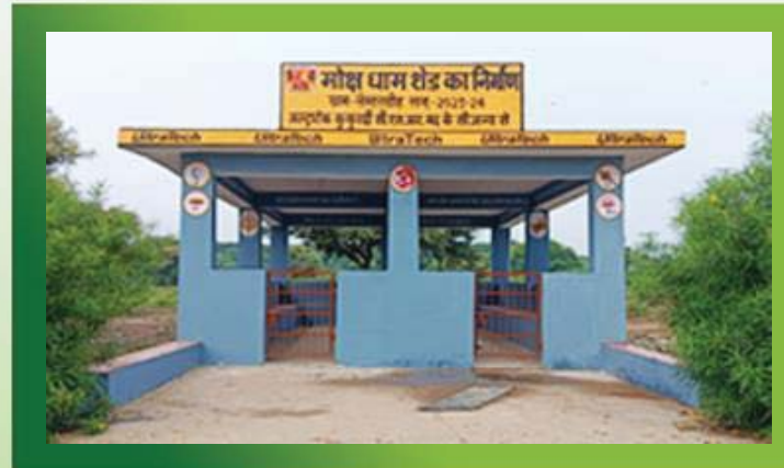
Kukurdihi Cement Works, Chhatishgarh
