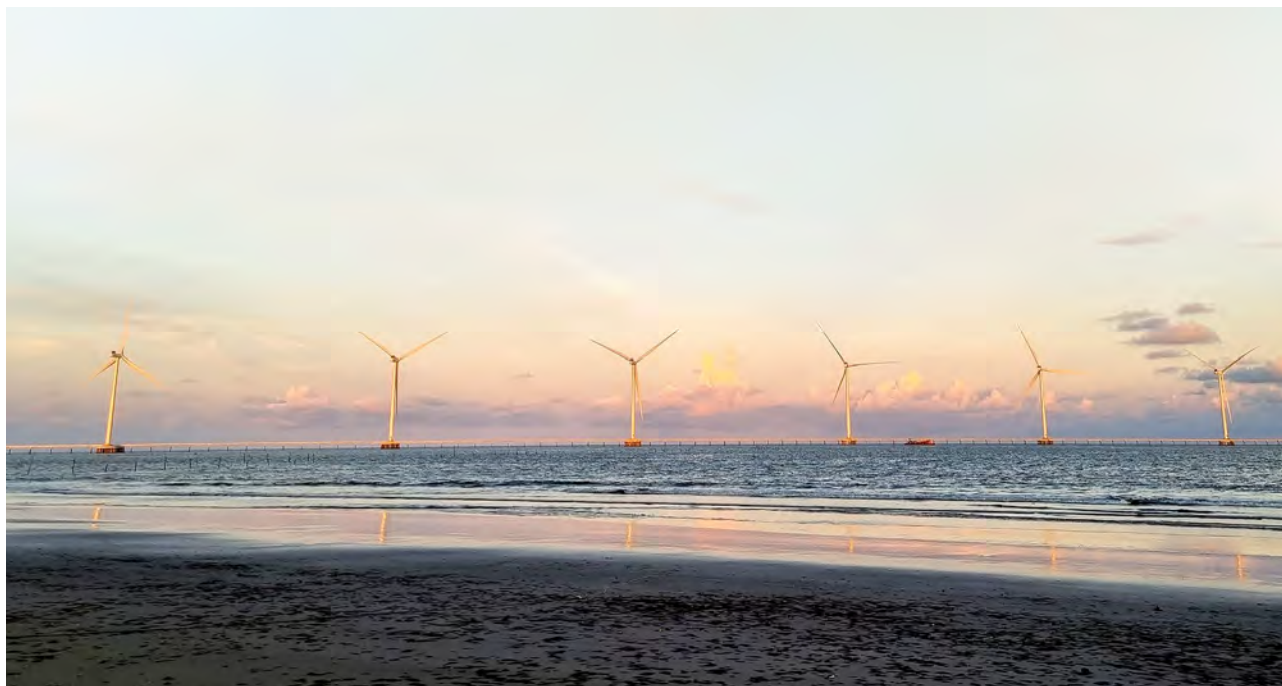
REE's Tra Vinh V1-3 Wind Power Plant
