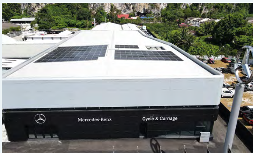
Rooftop solar at Cycle & Carriage Bintang Ipoh
