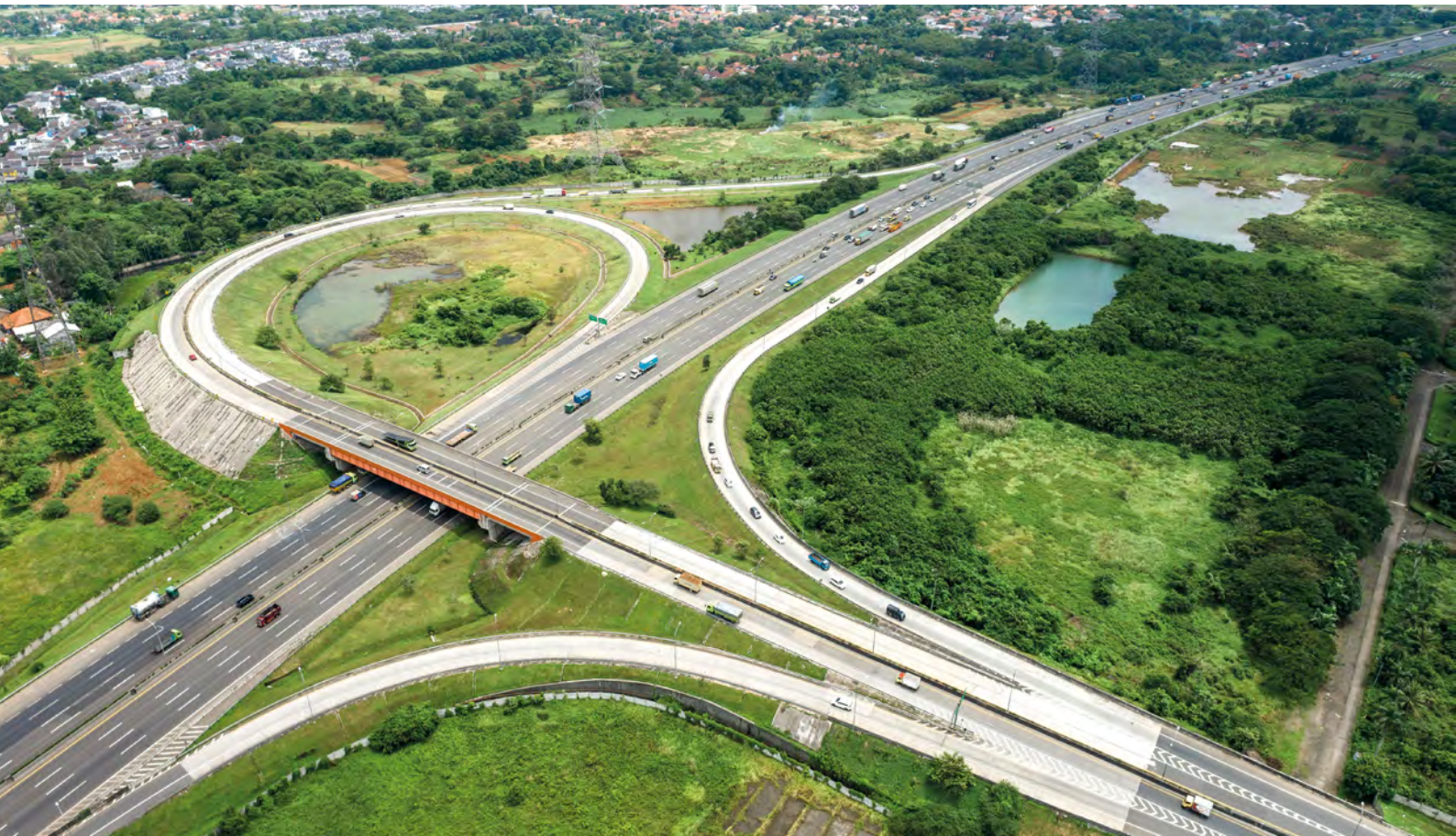
Astra's toll roads project on the Trans-Java network
