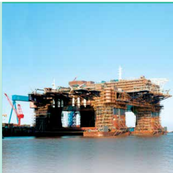
N503 An Xun 2 Semi-submersible accommodation vessel
