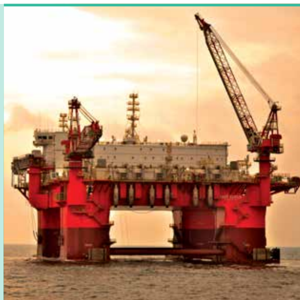
Safe Euros Advanced semi-submersible accommodation vessel
