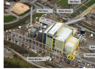
Wilton 11 (49MW or 190tph steam) 95% complete COD: 2H2016
