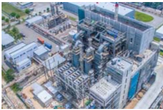
EfW Facility (140tph steam) 82% complete COD: 4Q2016
