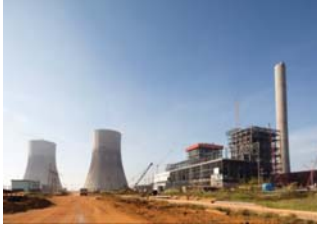
Semcorp Gayatri Power (1,320MW) 94% complete COD: 3Q2016 (Unit 1) 4Q2016 (Unit 2)
