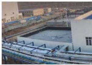
Changzhi TWMP (1.3 million m 3 /day) 82% complete COD: end-2016/2017
