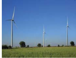
Semcorp Green Infra Rojwas (60MW) 100% complete
