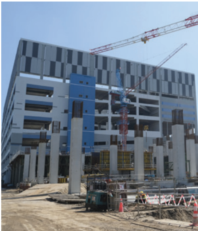
Jurong Island Logistics Hub Phase 2
