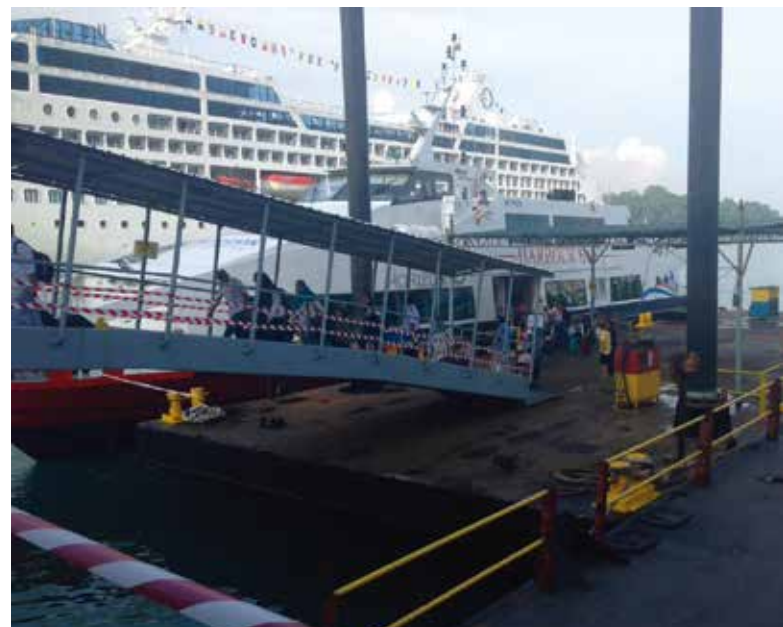
Construction of Temporary Floating Jetty for SG Cruise Centre's facilities
