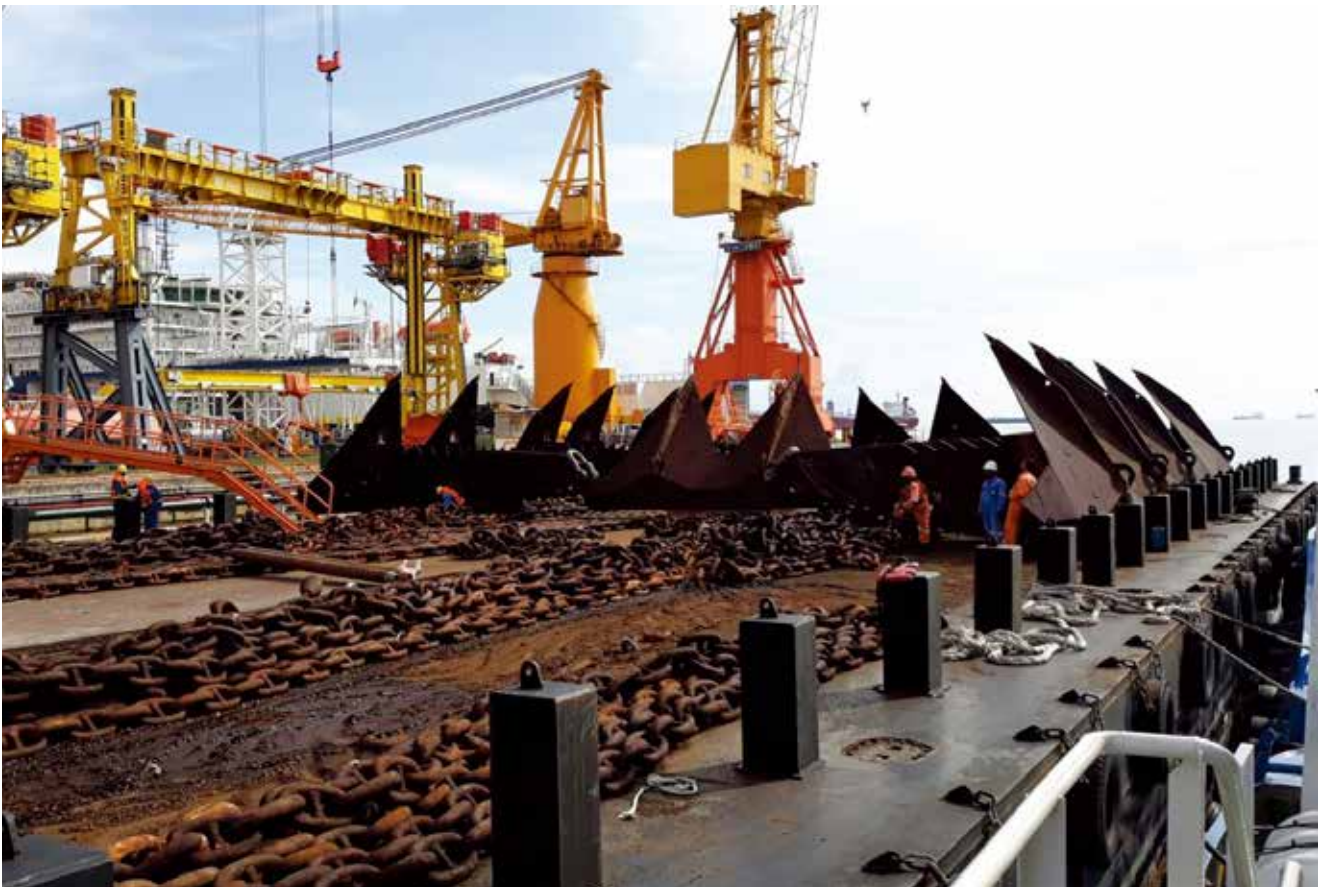
Heavy lifting of Anchor & Chains
