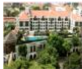
Village Residence Clarke Quay
