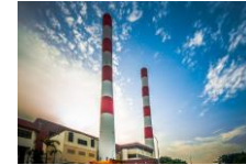
Senoko Waste-to-Energy (WTE) Plant
