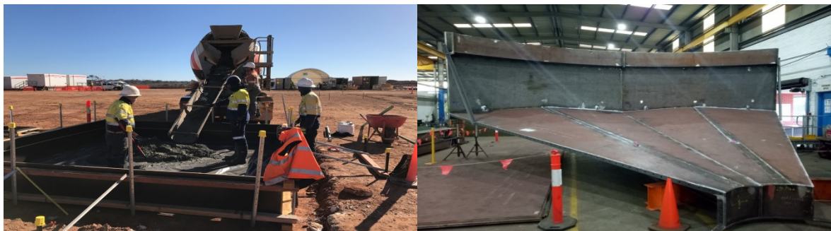
Figure 4 & 5 | First concrete pour - take up tower curing (left) and thickener fabrication progress - trial assembly of first two pie sections (right)
