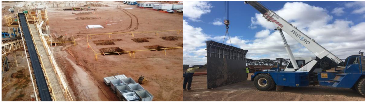
Figure 2 & 3 | Excavations for foundations (left) and cast in bar & shutter fabrication (right)
