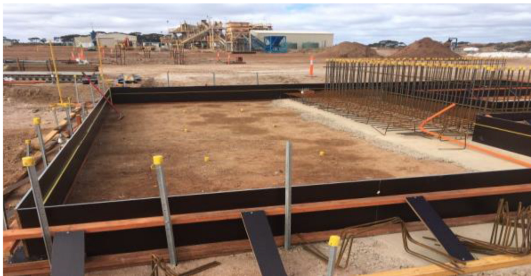
Figure 1 | Feed bin slab on north-end ready for blinding
