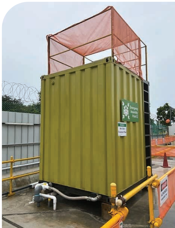
Biofuel specific membrane bio-reactor installed at a construction site.
