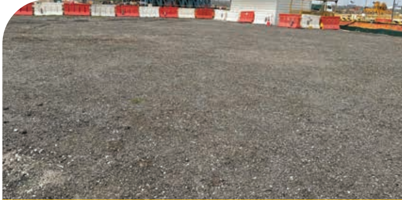
Re-use of mill waste to prevent soil erosion
