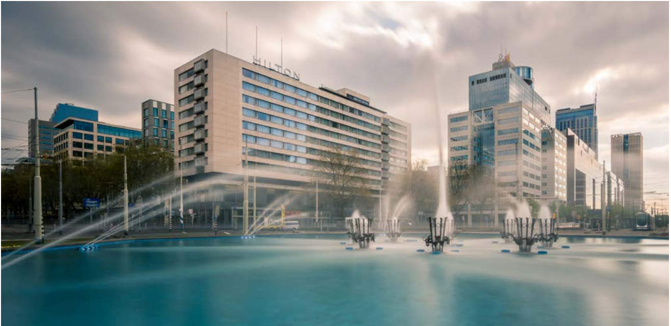
Hilton Rotterdam Hotel, Rotterdam, the Netherlands
