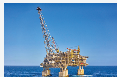
Wheatstone LNG Project, Australia Source: Chevron Australia
