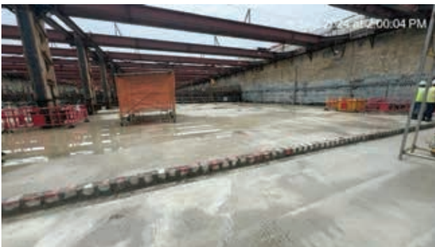
Concrete test cubes are re-used to build bund walls and sump tanks.
