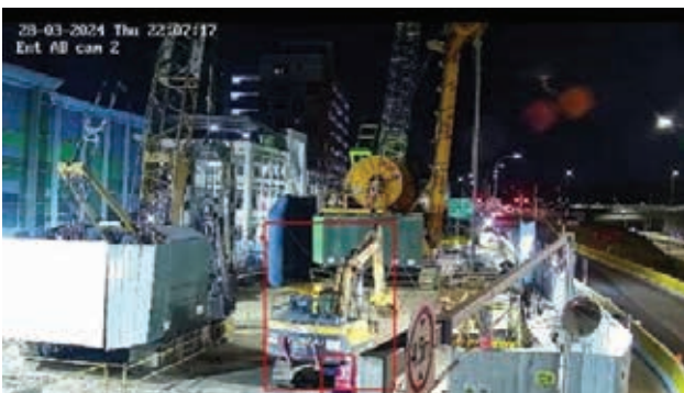
Video analytics is used to detect and flag personnel in close proximity of machineries.
