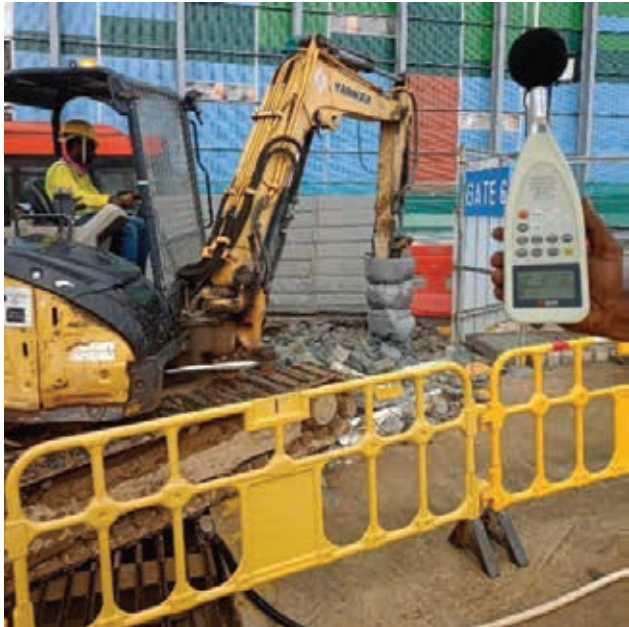
Noise barrier and padding were used for excavation works to reduce noise level.
