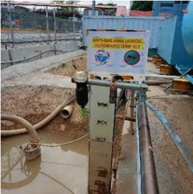
Anti-malaria oil automatic drip kit is used at our ECM ponds
