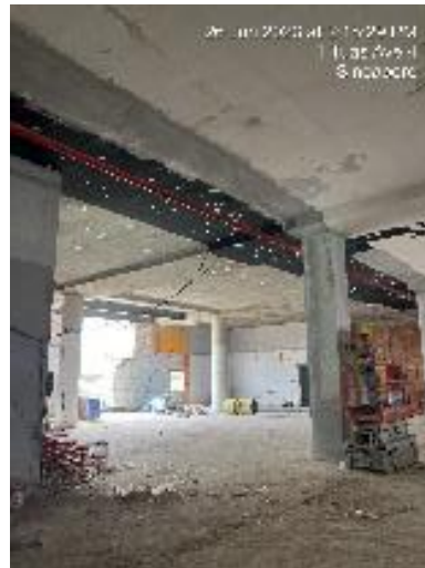
Touch Up Soffit of Slab @ L2
