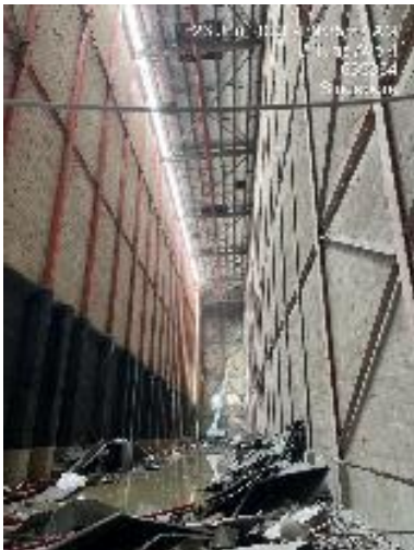
Removal of Existing Vermiculite
