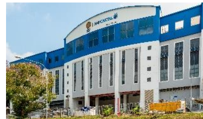
11 Changi South Street 3
