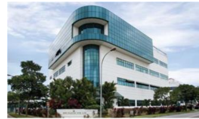
541 Yishun Industrial Park A
