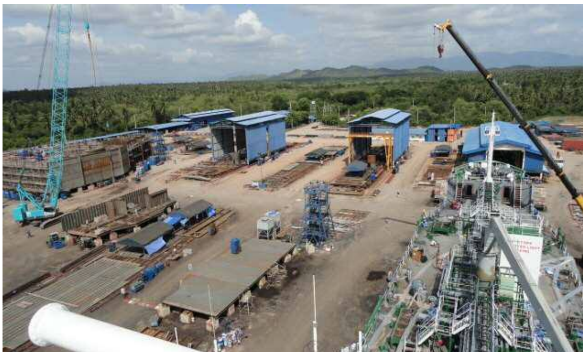
Left: Our shipyard in Thapsakae, Thailand, with 70,000 sqm of land space to undertake EPC projects and provide new building services such as offshore modules and oil rigs structures. We have successfully completed two EPC projects in this shipyard, and have successfully launched and delivered them to our customers.
