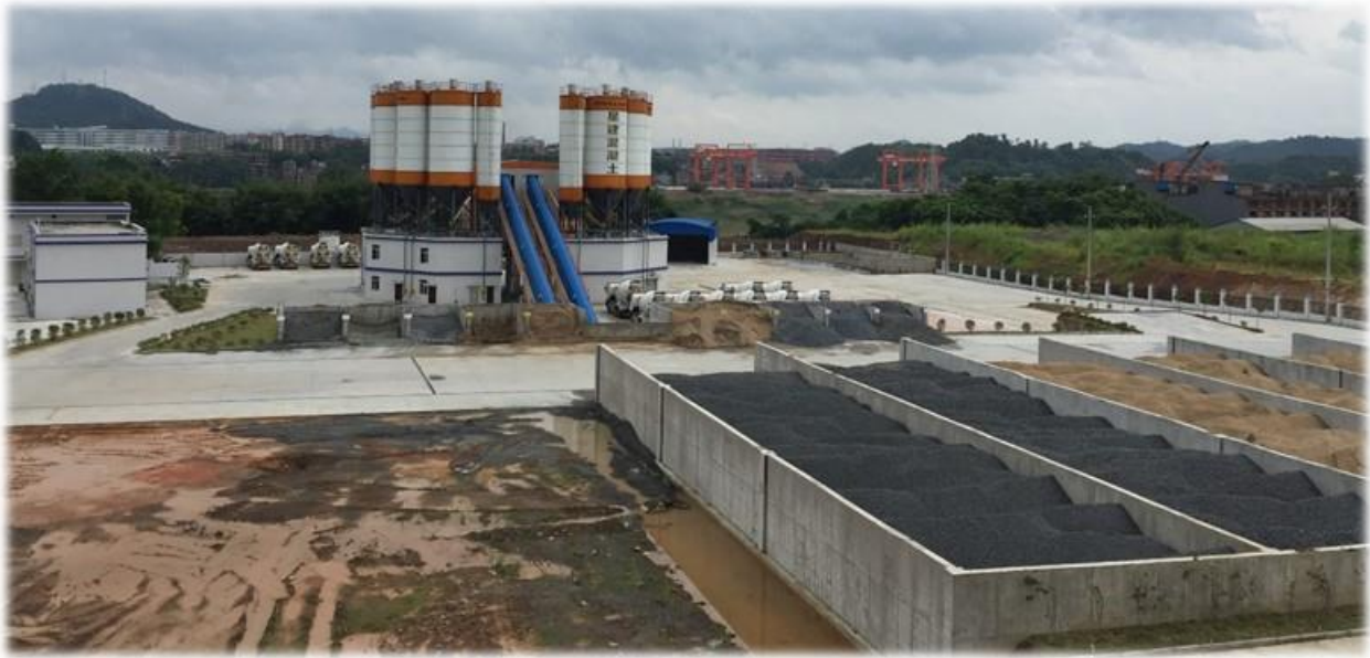
Wuzhou Xing Jian Ready-mix Concrete Manufacturing Facility
