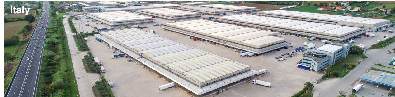
CLOM (Centro Logistico Orlando Marconi), Monteprandone - occupancy rate now at 99.9%:
