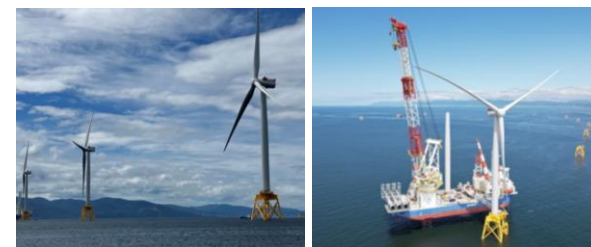
Turbine Generator Installation
