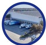
27-43 Toll Drive, Altona North
