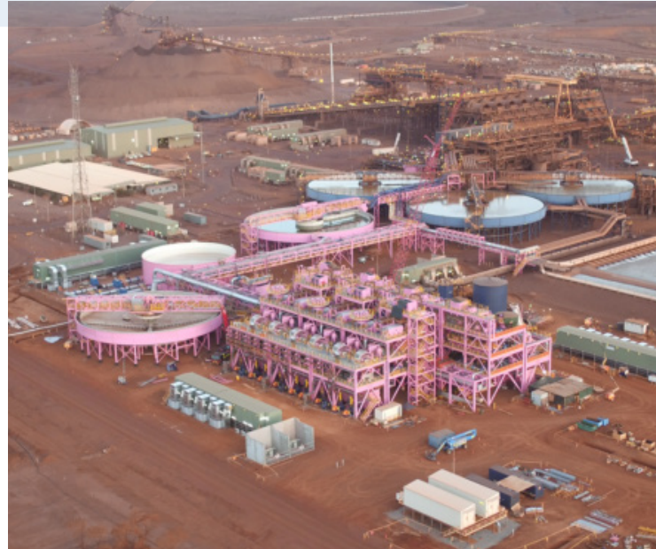
Roy Hill WHIMS Expansion - Greenfield Construction Package
