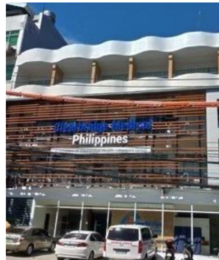
4-storey medical centre
