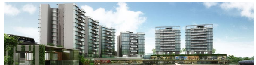
Watertown and Waterway Point
