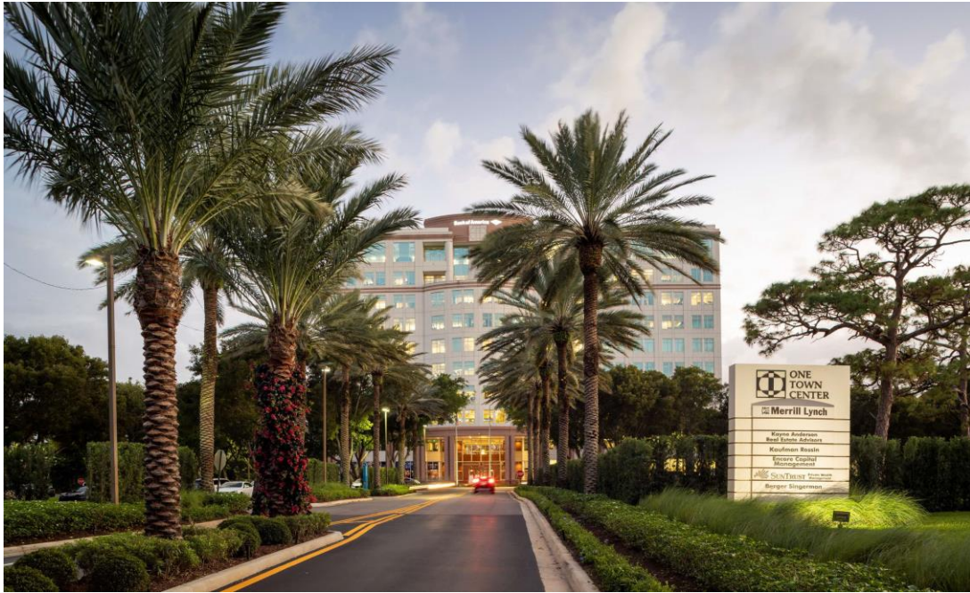
Figure 2. Front view of One Town Center
