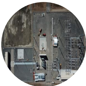
226MW Murra Warra Wind Farm Stage 1 completed FY20
