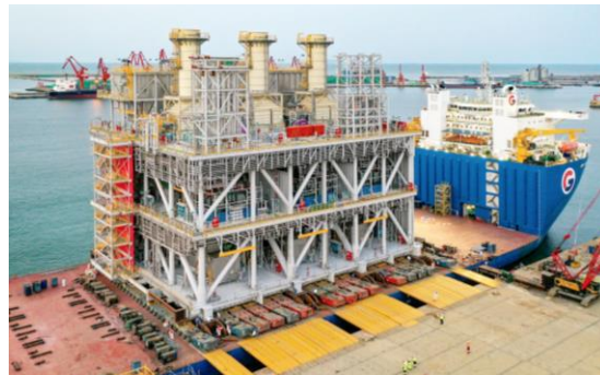
Waste Heat Recovery Units
