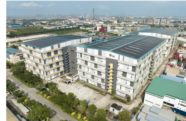
Solar panel installation at 20 Gul Way, Singapore
