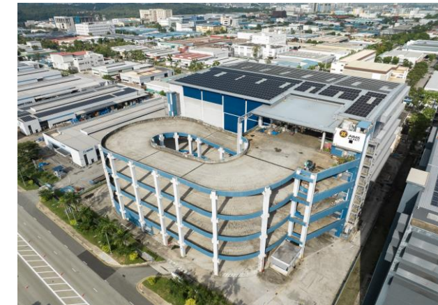
Solar panel installation at 30 Tuas West Road, Singapore
