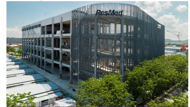
3 Tuas Avenue 2, Singapore
