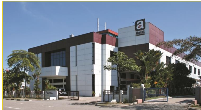
26 Tuas Avenue 7, Singapore
