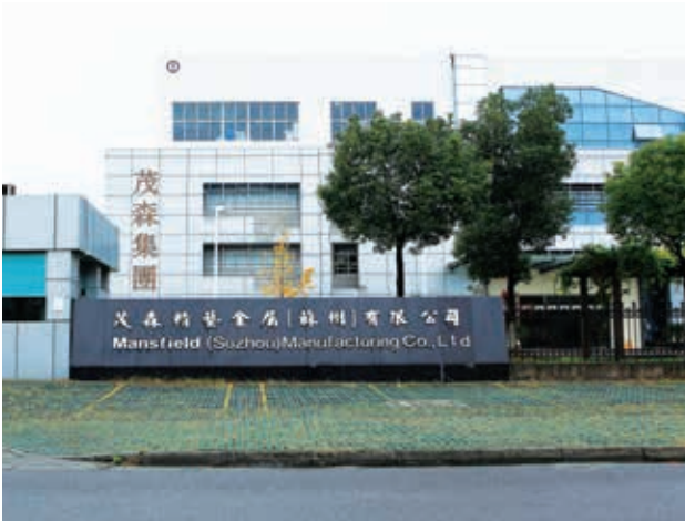
Mansfield Suzhou Plant
