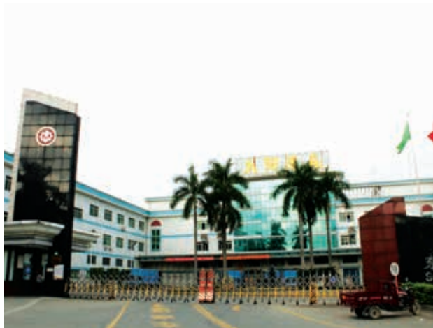
Sun Mansfield Plant
