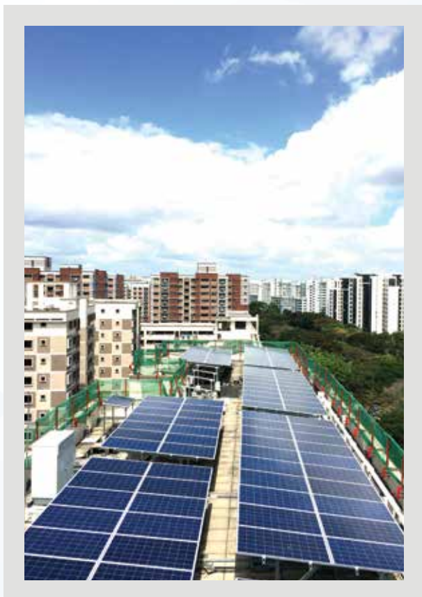
HDB SOLAR LEASING @ ANG MO KIO TOWN, SINGAPORE
