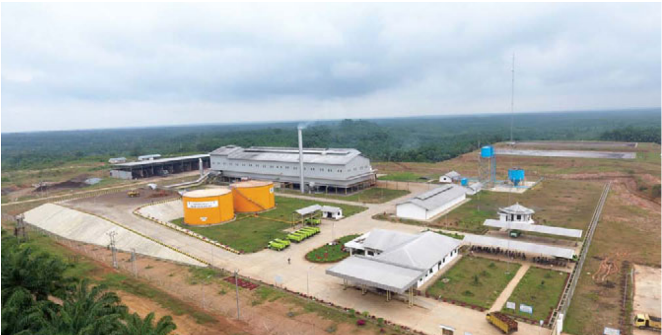
New Palm Oil Mill in South Sumatra
