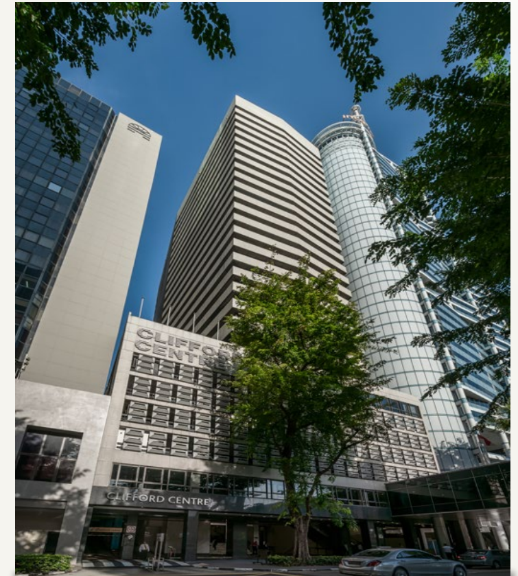
Clifford Centre is located adjacent to the Raffles Place MRT station.
