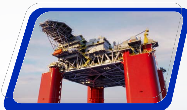
Tiber FPSU, the second Series Build unit awarded by bp, is based on more than 85% on Kaskida FPSU's design (shown above).
