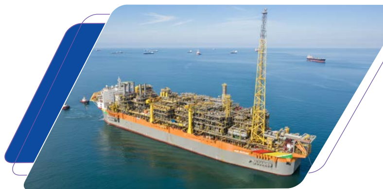
Successful delivery of One Guyana, Seatrium’s fourth FPSO project for Guyanese waters, to SBM Offshore after completing topsides fabrication, installation and integration.
