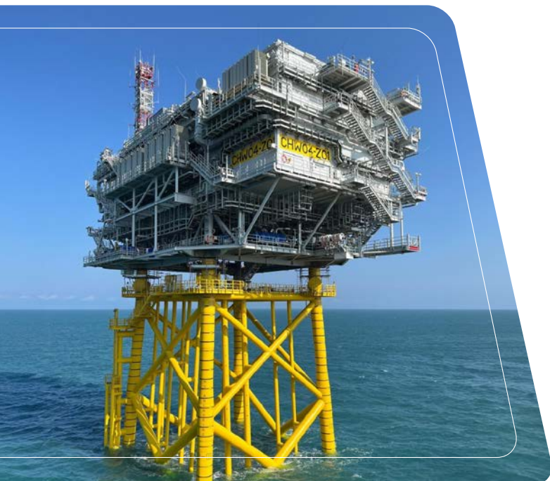
Completed delivery of Greater Changhua 2b and 4 Offshore Substation.
