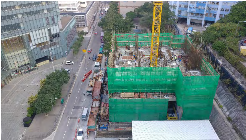
Existing site undergoing construction
