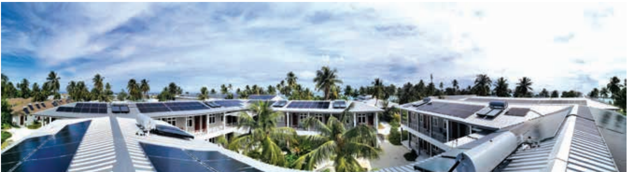
Solar panels installed at the Pullman Maldives Maamutaa Resort
