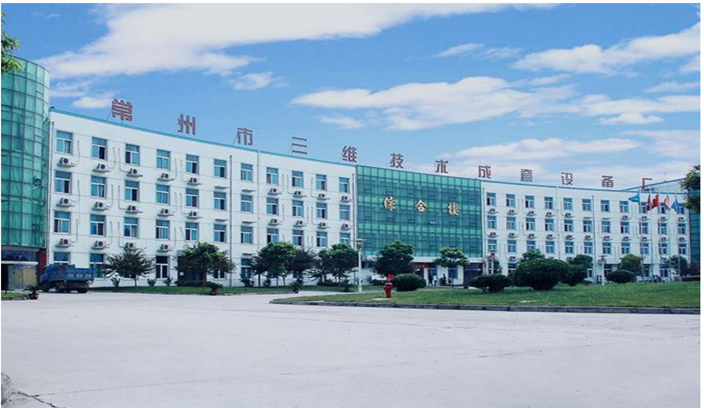
Figure 1. Main Building of Changzhou 3 D Technological Complete Set Equipment Co., Ltd, wholly owned subsidiary of STE
