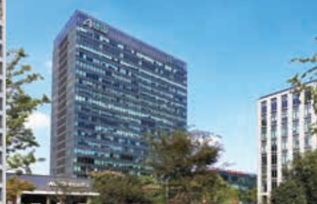
SINGAPORE-HANGZHOU SCIENCE & TECHNOLOGY PARK PHASE I
