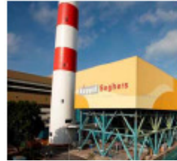
Tuas Waste to Energy DBOO Plant
