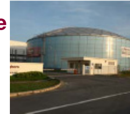
Ulu Pandan NEWater Plant
