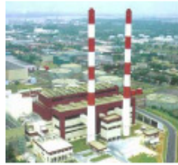
Senoko Waste to Energy Plant
