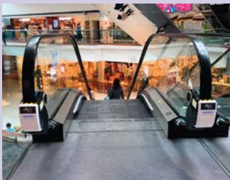
UV sterilisers in use on escalator handrails at Festival Walk mall.
