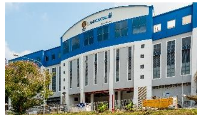
11 Changi South Street 3
