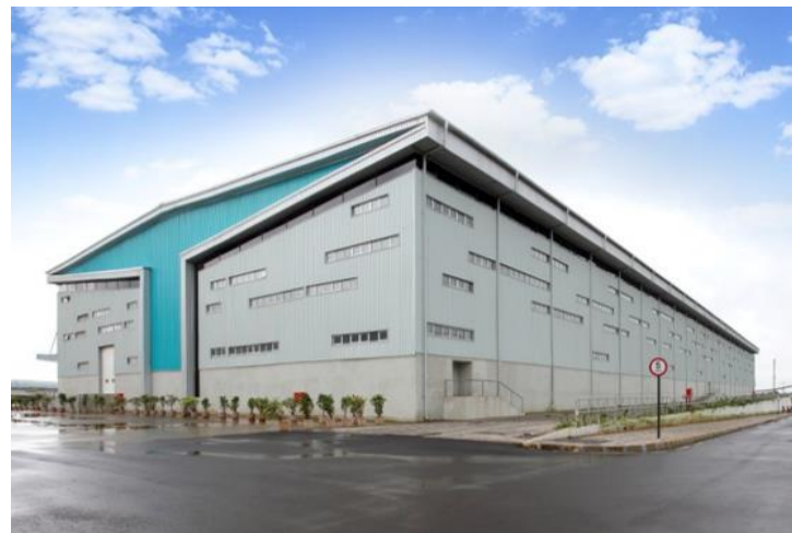
Arshiya Panvel Warehouses, Mumbai
