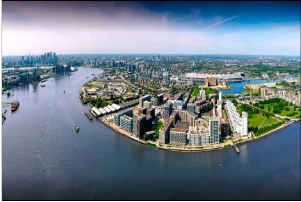
TOWNSHIP DEVELOPMENT Royal Wharf
