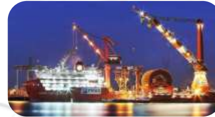
Installation of Multi-layer System (“MLS”)
