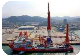
Installation of Huisman crane
