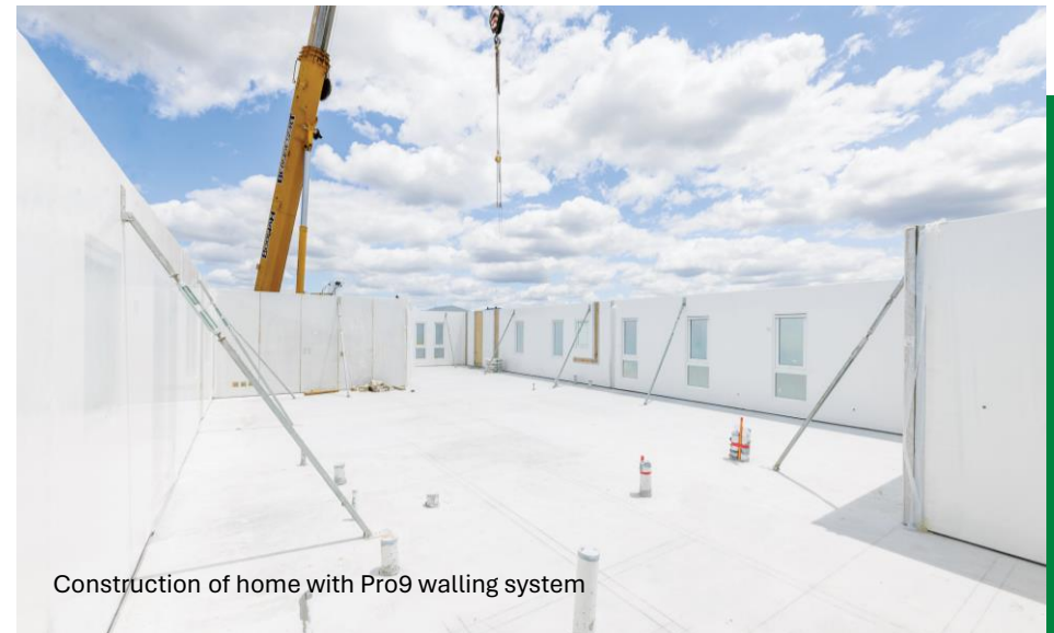
Pro9 walling being installed for a Stellar Collection home at Riverton, Jimboomba
