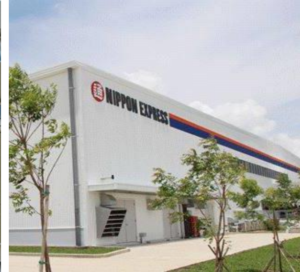
Industrial project at Thilawa Special Economic Zone
